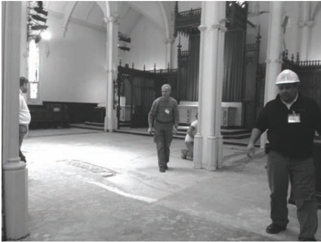
After the platforms were removed.
